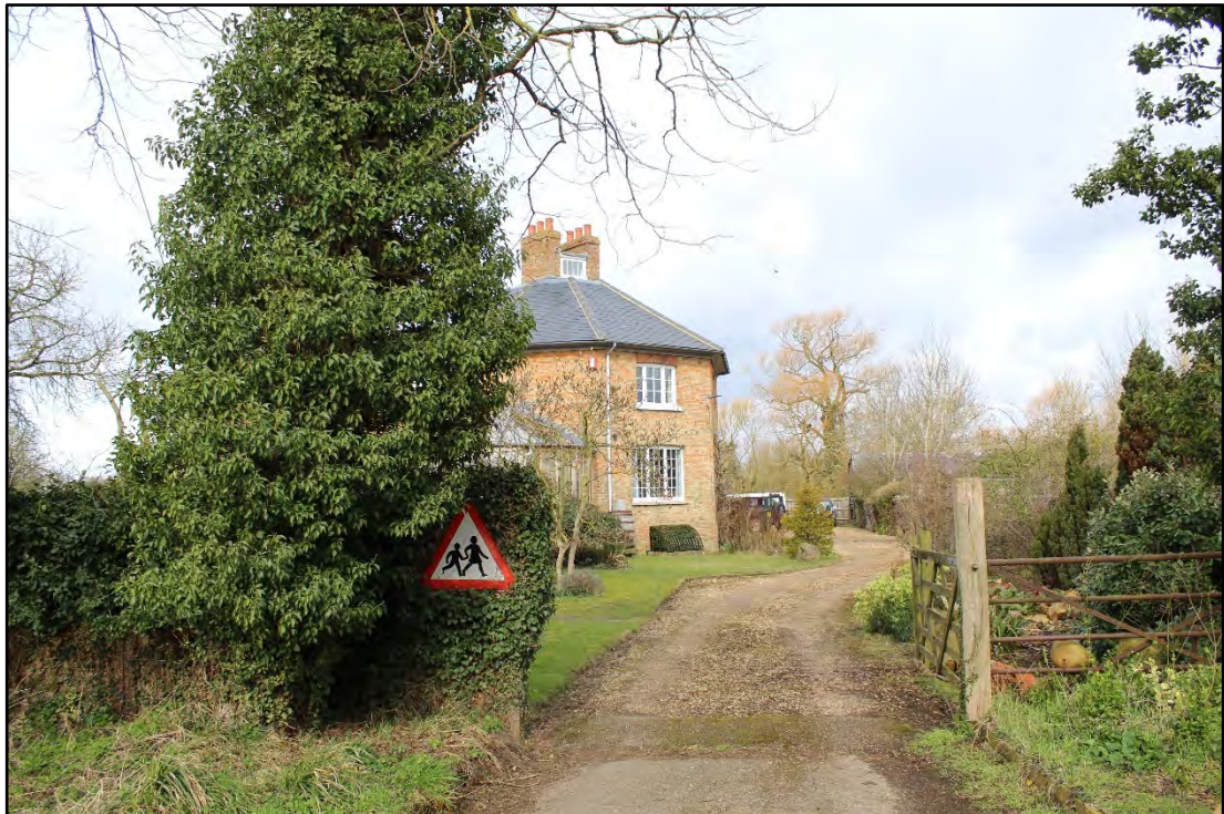
Photograph 1. Octagon Farmhouse, taken from the driveway to the farm, looking north west.
