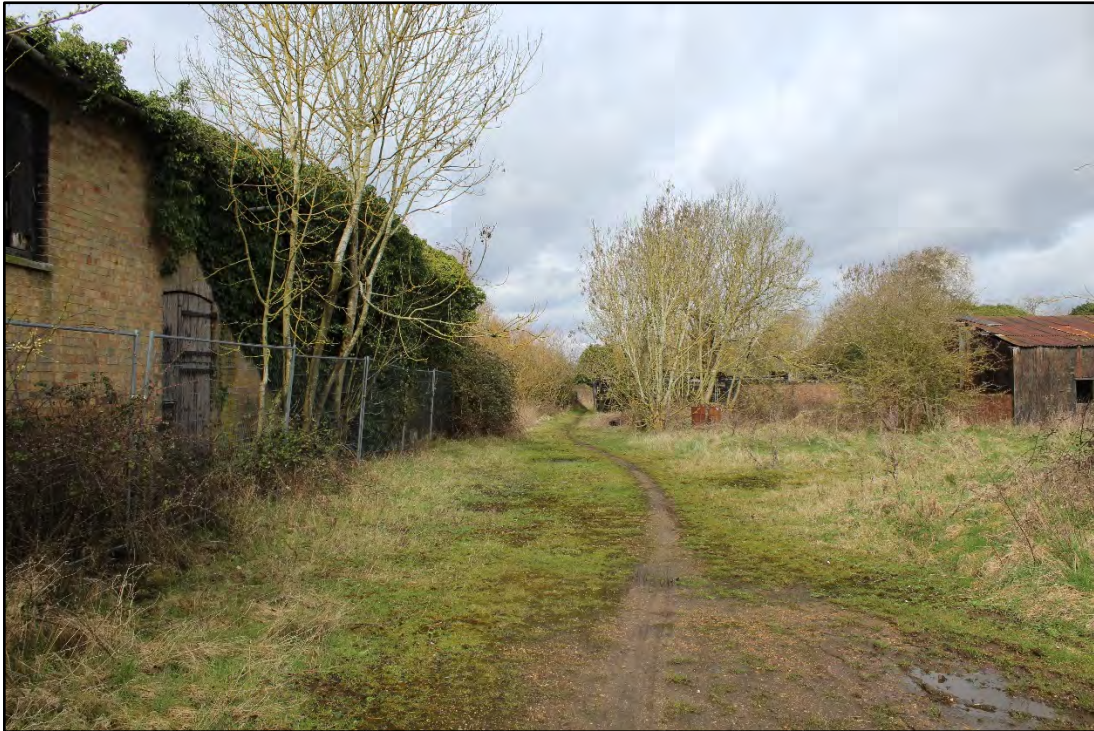
Photograph 2. Derelict farm buildings.
