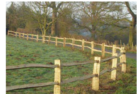
Post and rail fencing
