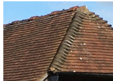
Roof tiles/ barn hip roof
