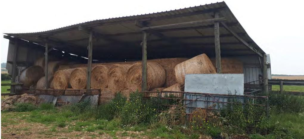
**Photo 1.** Building 1, photo facing west. Lean-to shed with corrugated steel cladding, used for hay bale storage (see Figure 2 for location).
