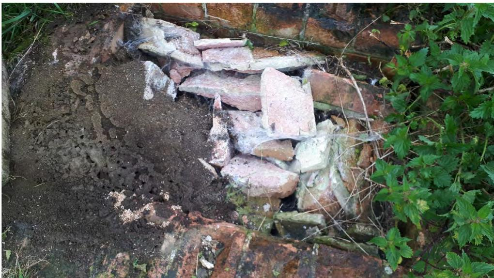
**Photo 12.** Abandoned drainage chamber filled in with rubble, located to south of farmyard (see Figure 2 for location).
