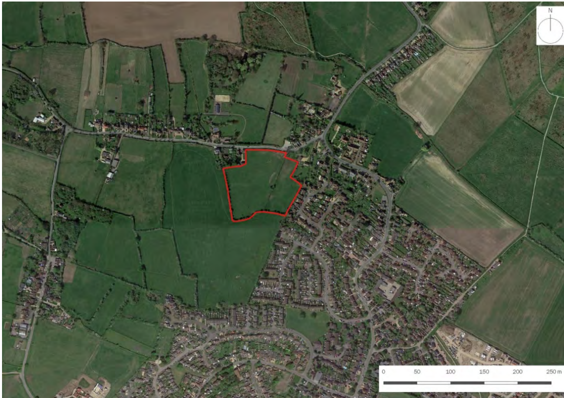
Image EDP 1: Aerial view of the site. Source: Google Map data 2021.
