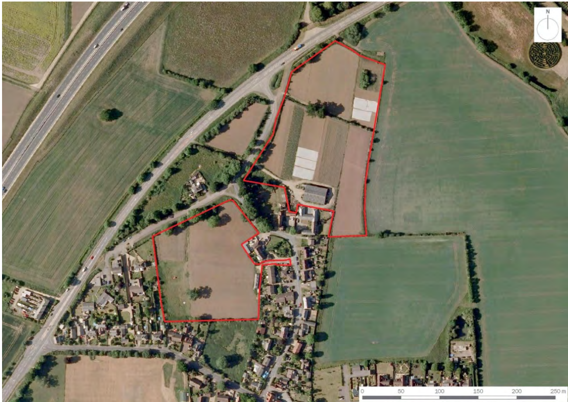
Image EDP 1.1: Aerial view of the site. Source: Google Map data 2021.
