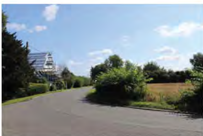
Fig.14. The Cottage as seen from Green End Road looking east
