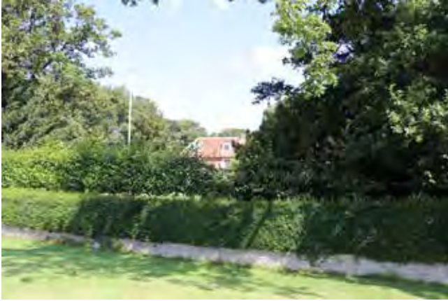
Fig. 10. Kempston House as seen from the south (access track to Ramsay Cottage)
