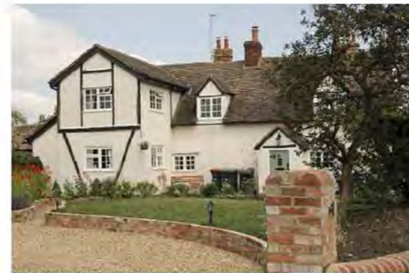
Off white cement render, timber frame and plain clay tiles
