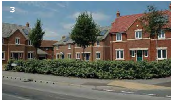
3 Brown and orange brick, dressed stone detailing
