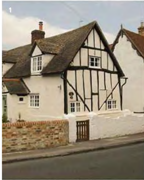
1 Timber frame give a more historic character and interest
