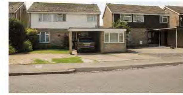
Yellow brick, tile hanging/pvcu fascia board, pantiles
