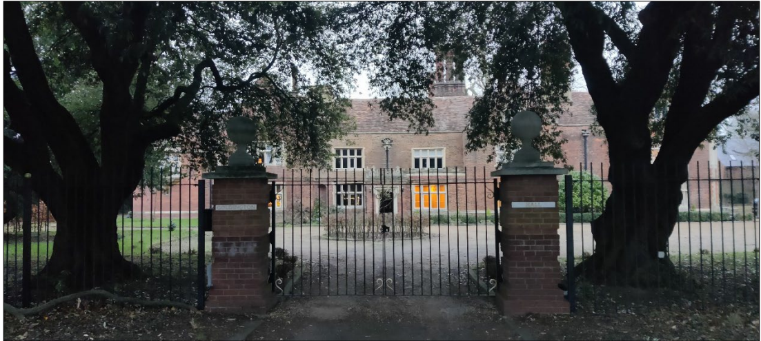
Photo 13 View of Goldington Hall front gates
