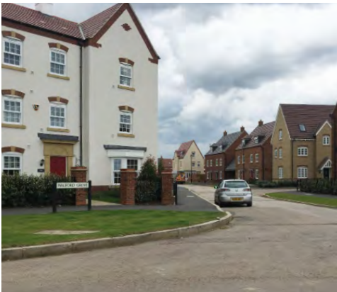
New housing at Kempston, east of the ring road
