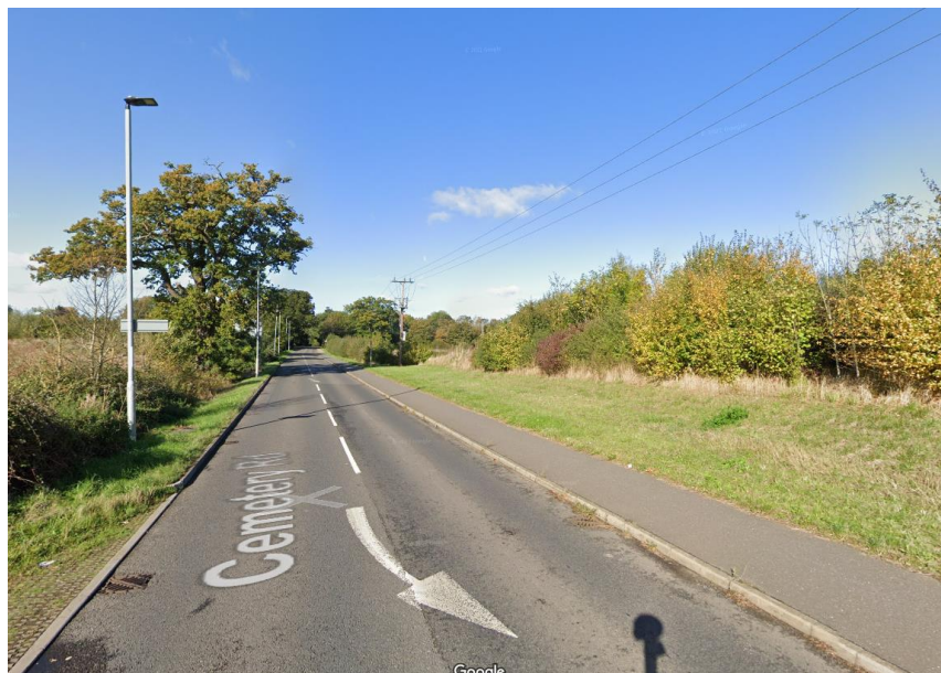
Figure 3.3 - Existing footway provision, Box End
