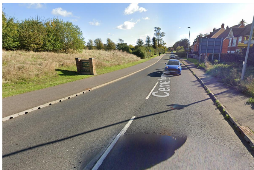
Figure 3.2 - Existing footway /cycleway, Cemetery Road
