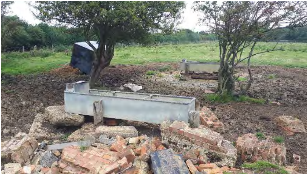
Photo 13. Rubble pile and troughs to north of farmyard, photo facing north. Scrapped water tank visible in left rear ground, sitting in hole left by landowner while decommissioning mains water supply to troughs (see Figure 3 for location).
