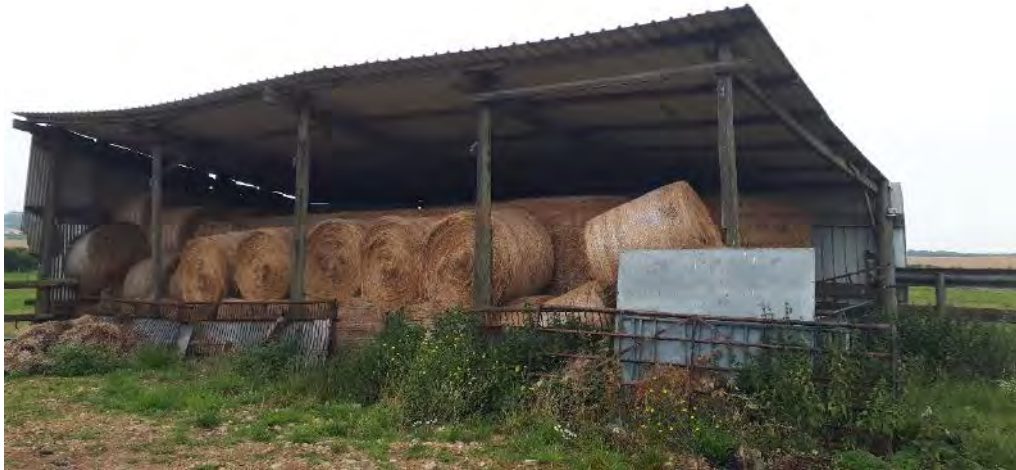
Photo 1. Building 1, photo facing west. Lean-to shed with corrugated steel cladding, used for hay bale storage (see Figure 2 for location).
