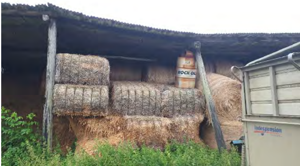
Photo 2. Building 2, photo facing south. Lean-to shed with corrugated cement cladding, used for hay bale storage. Empty oil drum used as support. (see Figure 2 for location).
