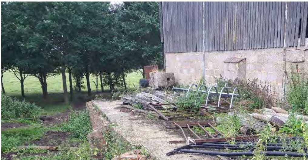
Photo 8. Location of former diesel tank east of Building 3, photo facing south. Brick retaining wall below concrete hardstanding. Empty oil drum and stack of corrugated cement sheeting in centre of photo (see Figure 3 for location).
