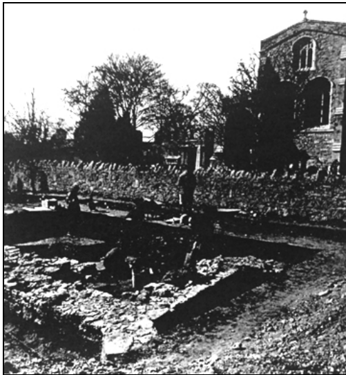
Figure 4. Excavation to the east of the churchyard wall (Baker, 1968)
