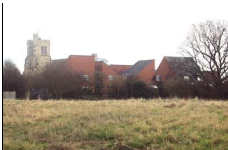
Figure 46. The steeply pitched roofs of Abbey Close viewed from the west
