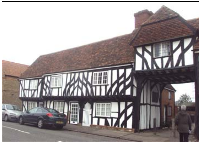
Figure 31. Decorative timber bracing to nos. 1 – 3 Bunyan's Mead
