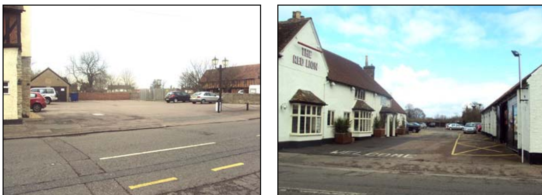
Figure 35. Large areas of hard standing adjacent to The Swan and The Red Lion
