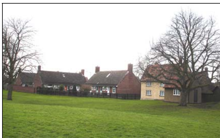
Figure 43. Housing on the north side of The Green
