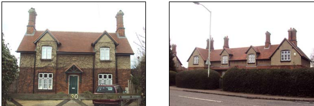
Figure 48. Examples of the estate cottages on the north side of West End, built in 1903
