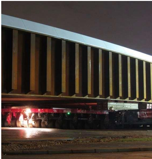
Figure 3.3: Leigh Road Bridge off line structure ready to be driven in
