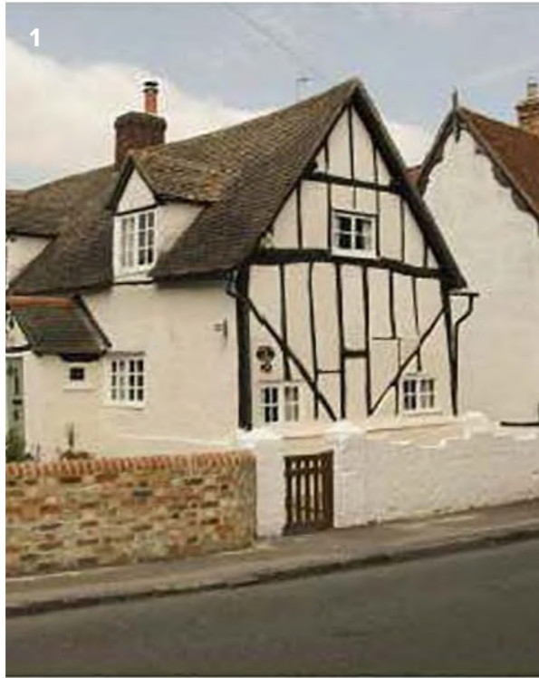
1 Timber frame give a more historic character and interest
