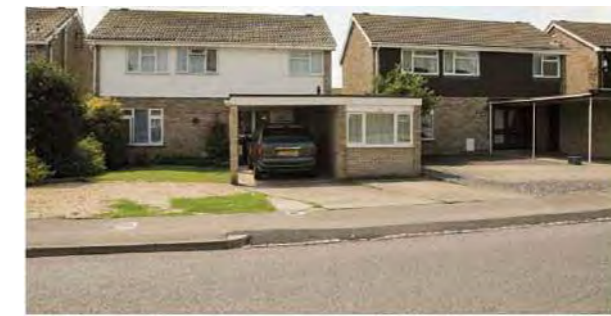
Yellow brick, tile hanging/pvcu fascia board, pantiles
