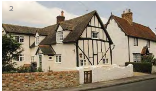
2 Timber frame, dormers, cement render and plain clay tiles
