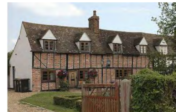
Structural timber frame with brick panels and clay tiles
