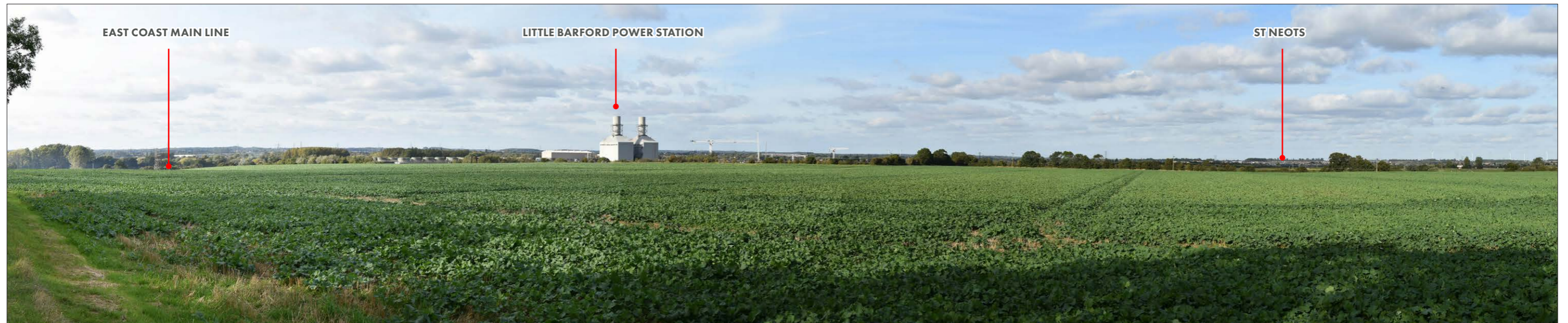
PHOTOGRAPH – VIEWPOINT S8: VIEW FROM THE NORTHERN FIELD BOUNDARY WITHIN THE EASTERN PART OF THE SITE, LOOKING NORTH TOWARDS LITTLE BARFORD POWER STATION AND ST NEOTS.
