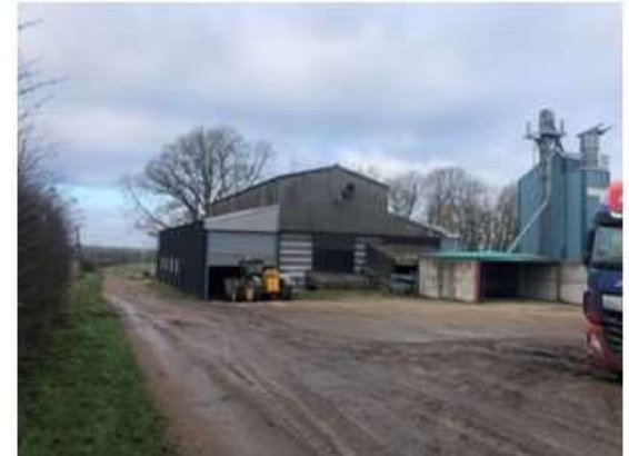
Photo 21: Building 2 (R) and 3 (L)
