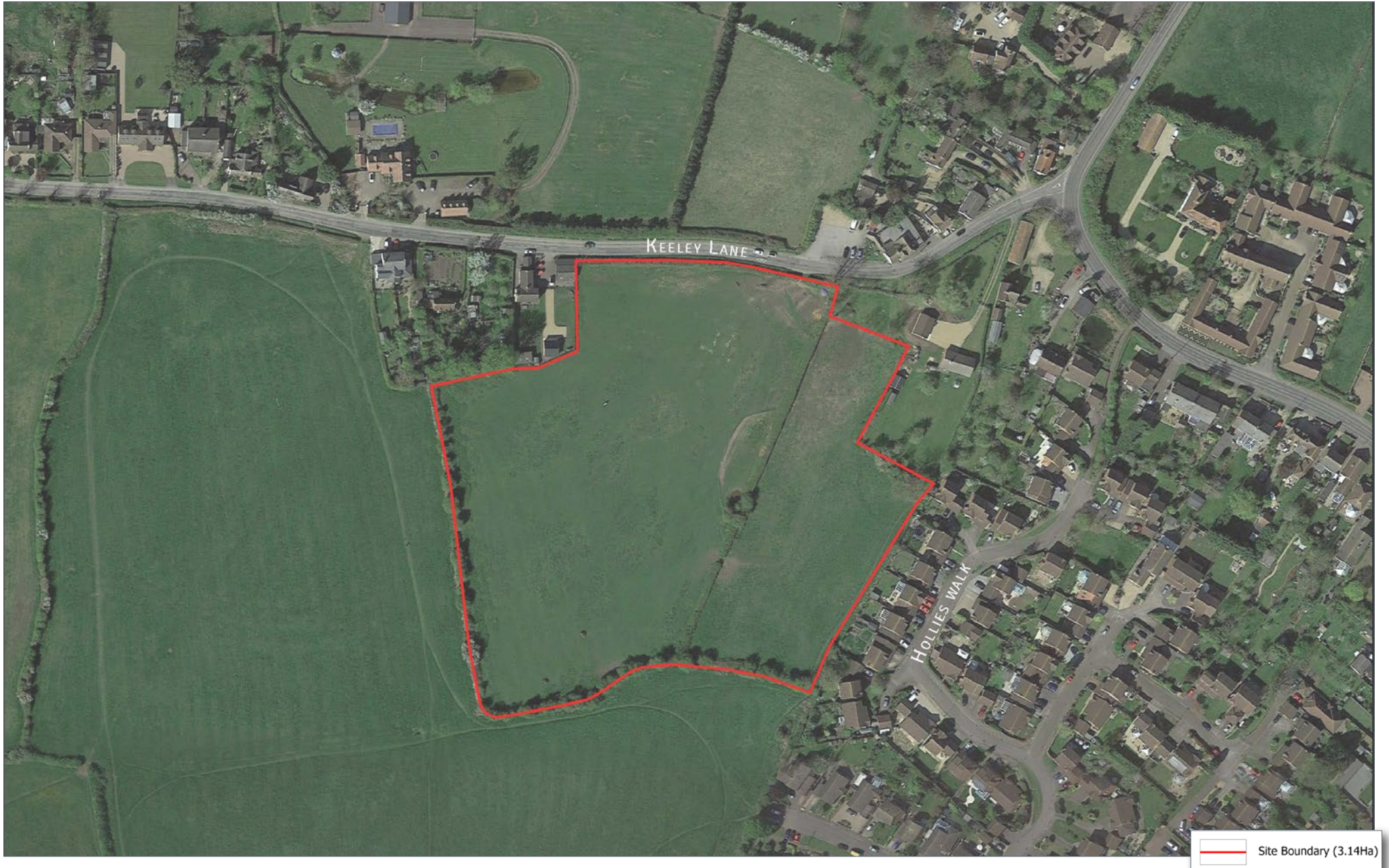
Aerial View of Site
