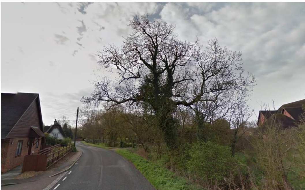
Plate 26: View towards northern gable end of No.35 Ravensden Road, with Abbey Close in foreground to left and Carlton House to right
