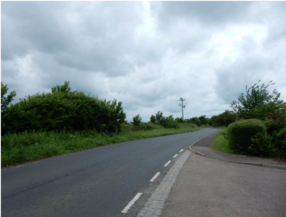
Plate 1: Eastern site boundary along Ravensden Road from the entrance to Abbey Close, looking north-west
