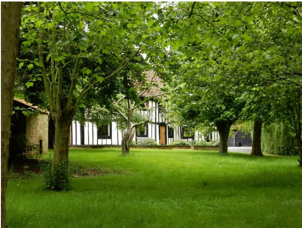
Plate 14: View north-west from eastern end of public footpath across garden towards front of Abbey Farmhouse
