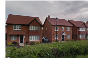
Red brick and clay tiles
