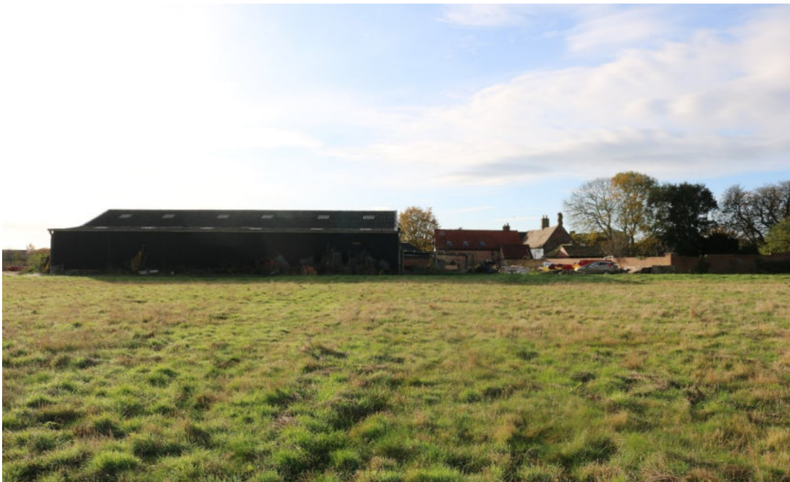
Image EDP 5.3: View from south of Parcel A, looking south toward modern farm barn and College Farmhouse (seen on right, building with chimney stacks).
