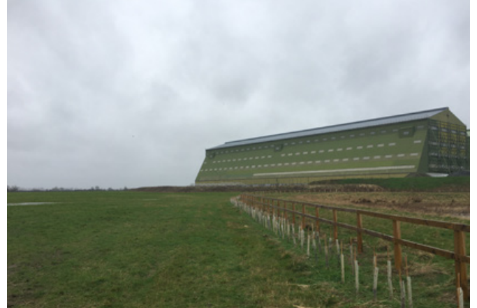
View of site from the east
