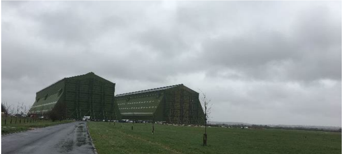
Figure 1: View looking east towards the western entrances of the sheds, taken from current entrance to the hangar site off A600
