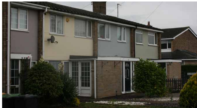
Figure 25: Housing on High Street
