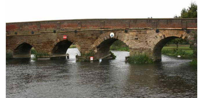
Figure 15: Barford Bridge Scheduled Monument
