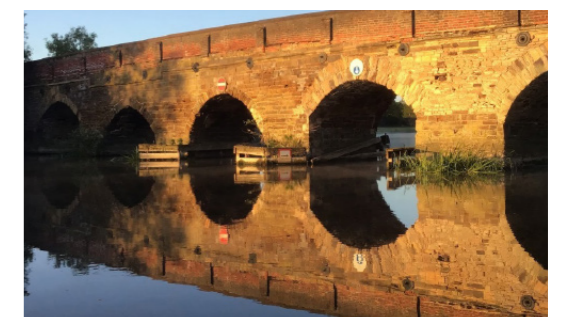
09 Great Barford Bridge
