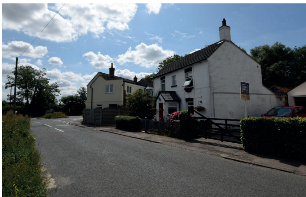
PHOTOGRAPHS ILLUSTRATING OLDER HAMLET DEVELOPMENT AT TINKERS CORNER A SHORT DISTANCE TO THE WEST OF THE PROPOSAL SITE
