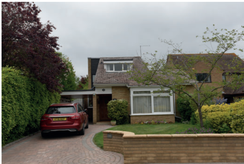
EXAMPLES OF 20th CENTURY SUBURBAN DEVELOPMENT IN CLOSE PROXIMITY TO LISTED BUILDING AT 39/41 CHURCH END, BIDDENHAM
