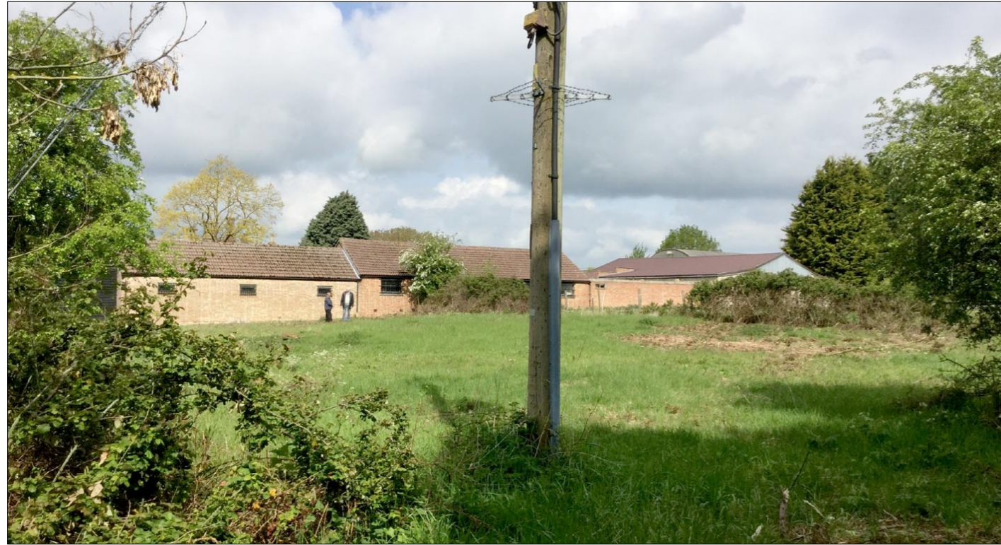
6. Overview of Application Site and Heddings Farm outbuildings, from SE.
