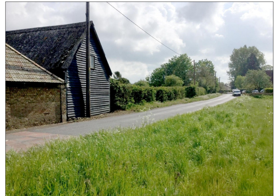
10. Road frontage view of Application Site on The Lane. Facing ENE
