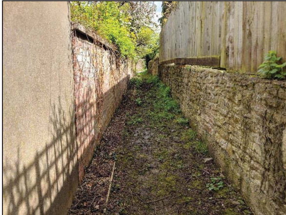
Figures 6 and 7: Conditions of Footpath 7
