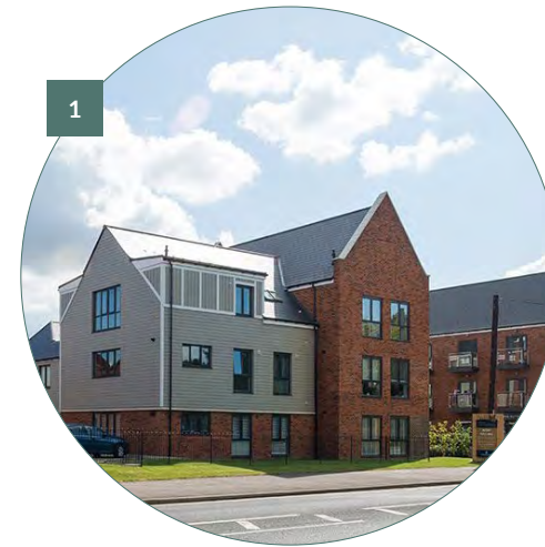
Example of apartments with gable walls and varied roofscapes and steps of building line. Image of Horstead Park, Courtesy of Clague Architects
