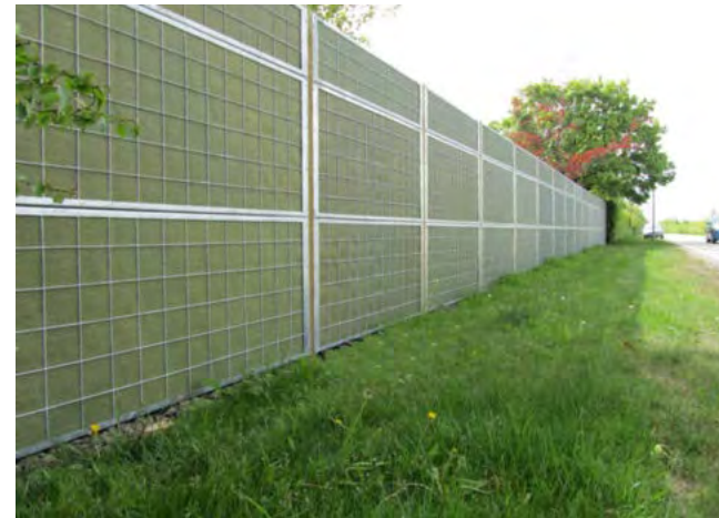
Example of green acoustic barrier
