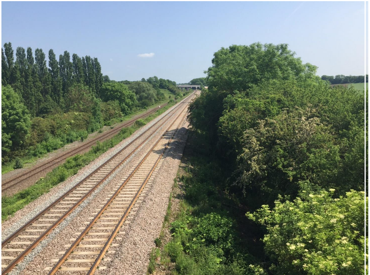
Figure 2-1 View of Slow Lines and Fast Lines
