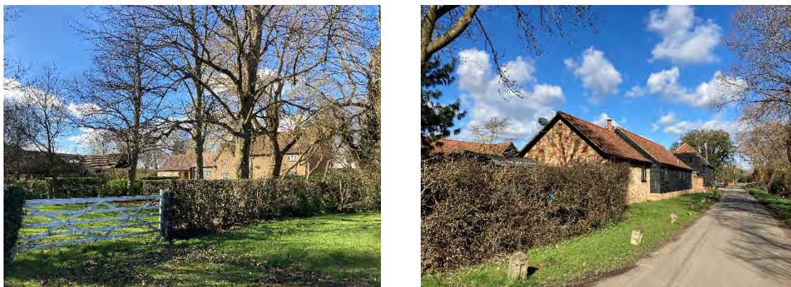
Figure 2 (L) Vicarage Farm; (R) Barn at Duck End Farm.
