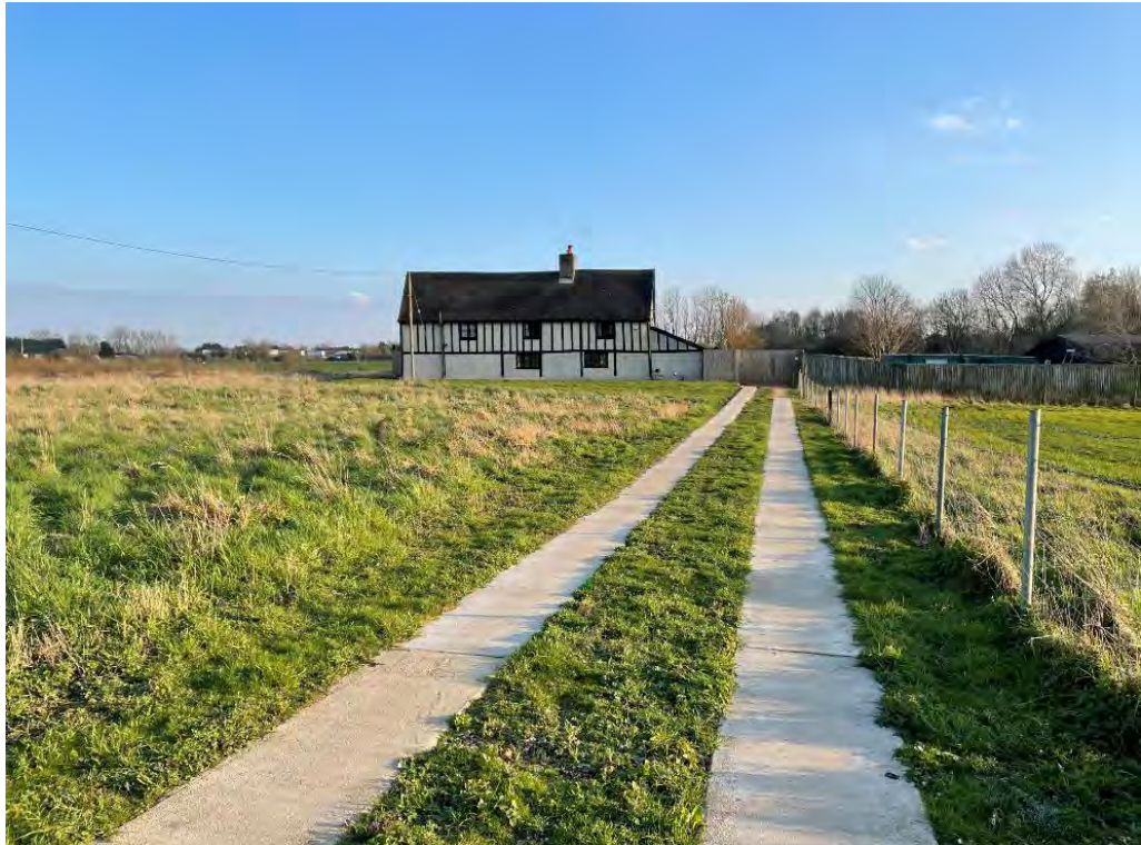
Plate 11: Moat Cottage, view to south
