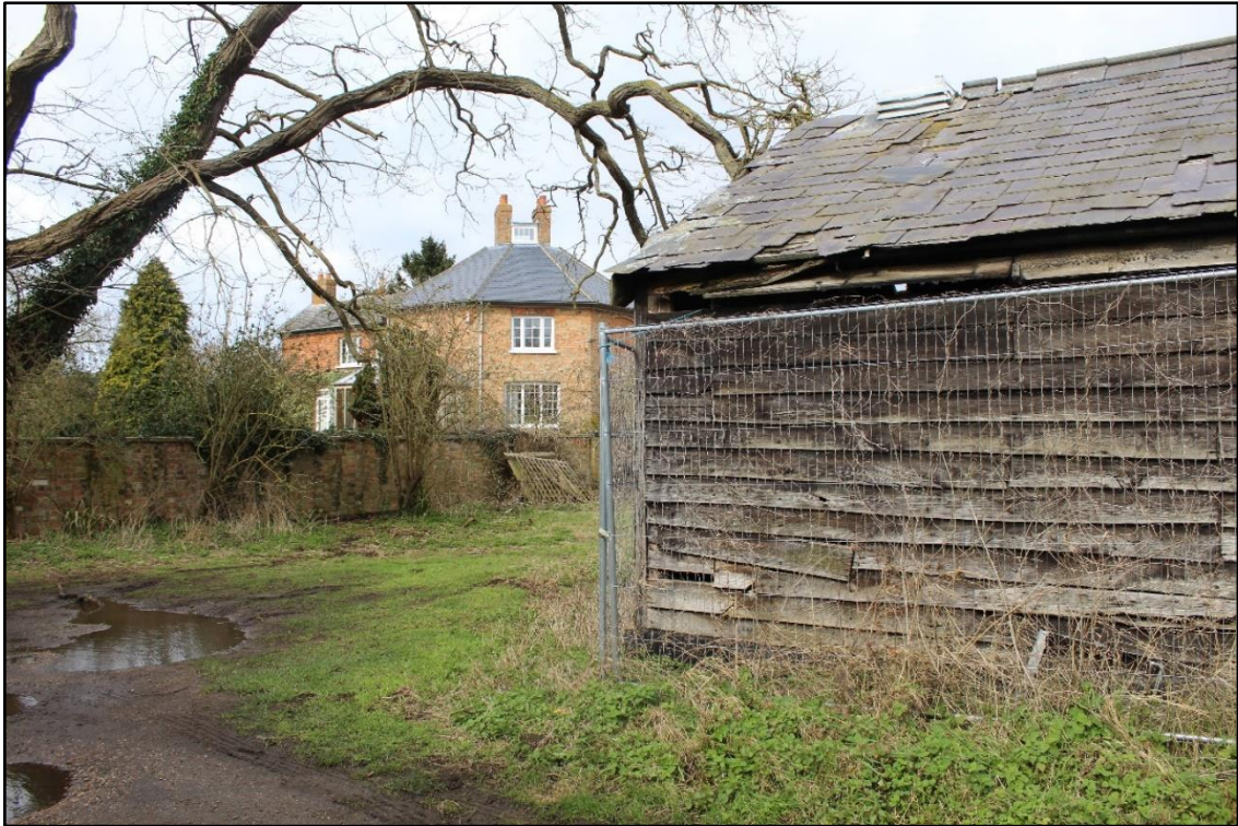
Photograph 4. Derelict farm building with Octagon Farmhouse in the background
