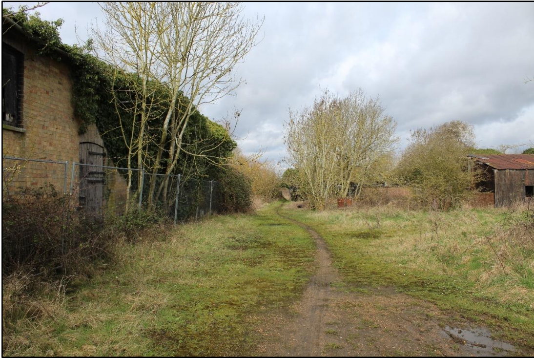
Photograph 2. Derelict farm buildings.
