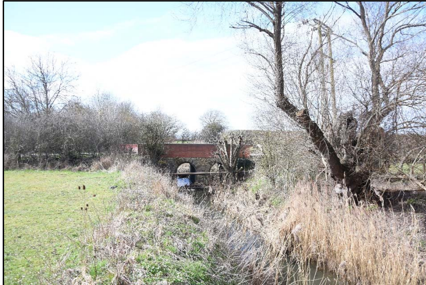
Non-designated heritage asset Hardwick bridge, looking south-west Fig 13
