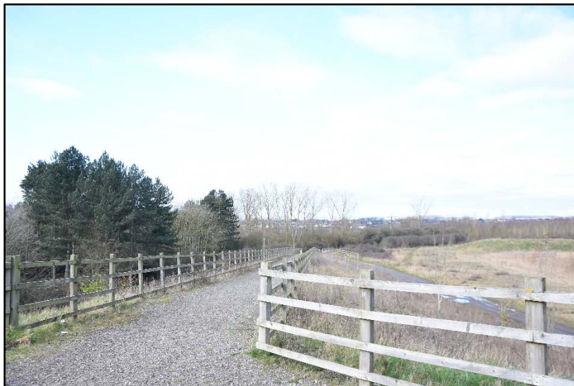
Area of disused medieval road that would have continued across this area towards Keeley Green, looking west Fig 67
