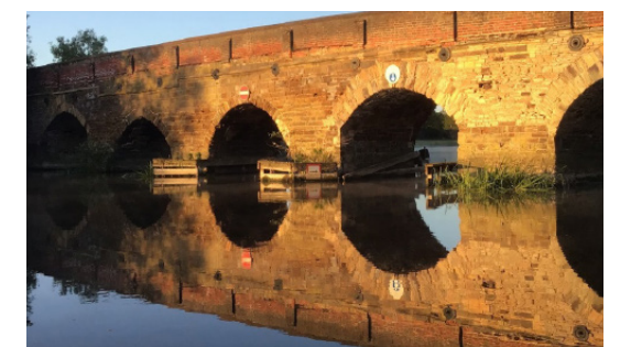
09 Great Barford Bridge
