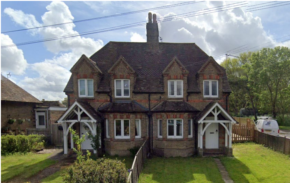
Figure 14 Nos 1-8 The Cottages
