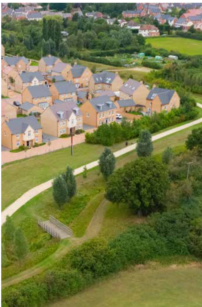
Fig.12 - Barratts Development at Wixams
