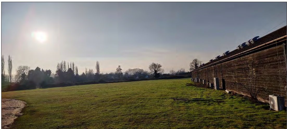
Photo 7 View of the Listed Buildings from south of the Site
