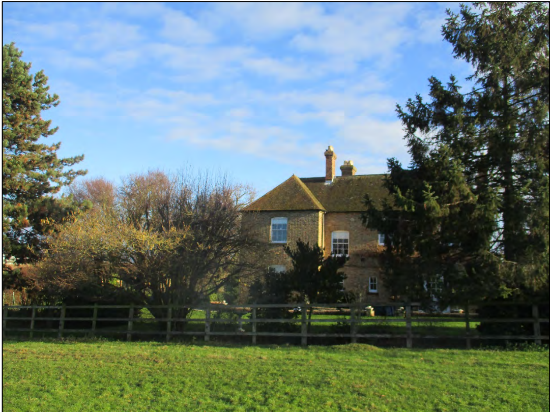
Photo 6 View of the western elevation of Harrowden House from within the Site
