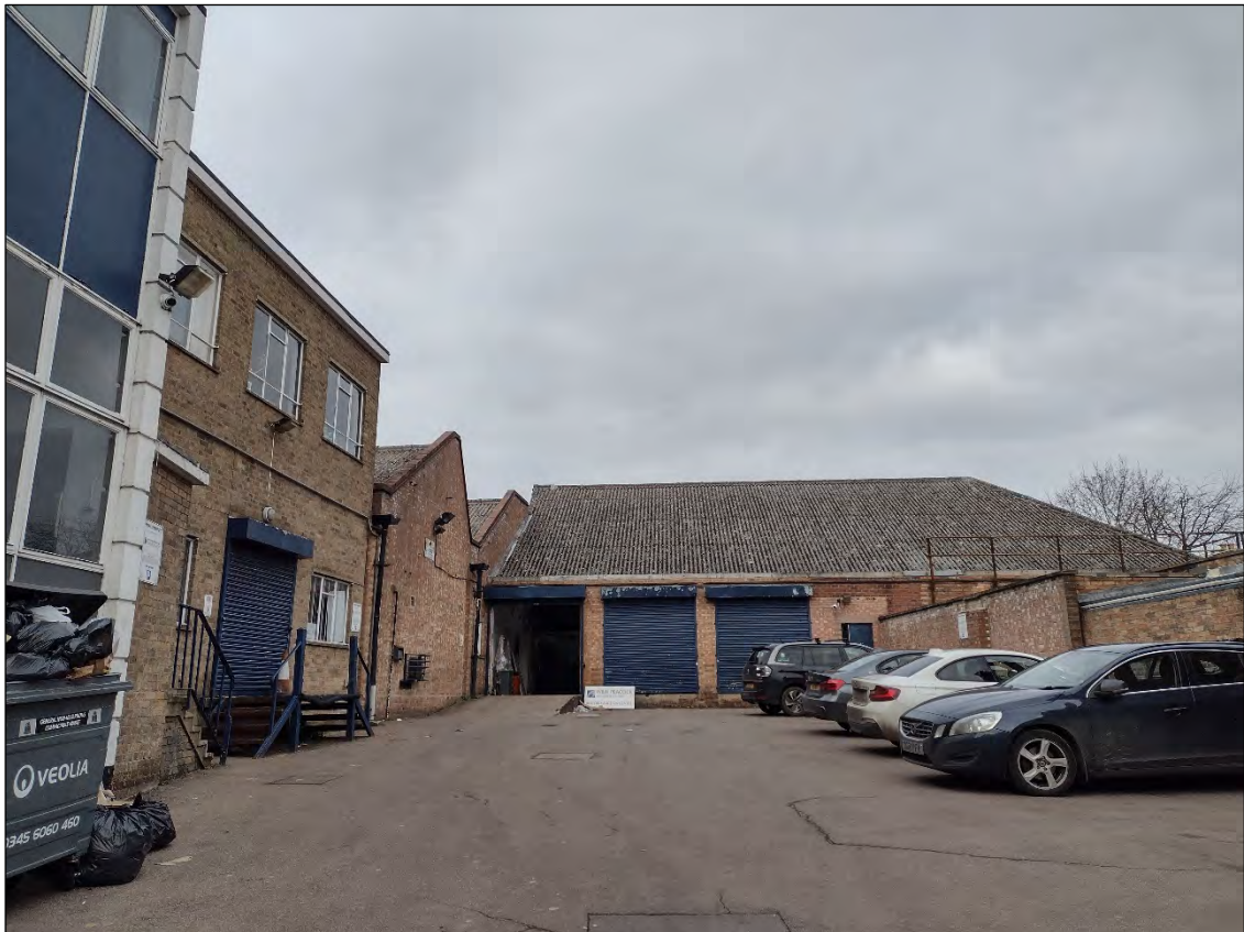
Photo 3 Auction buildings in the south-east of the Site
