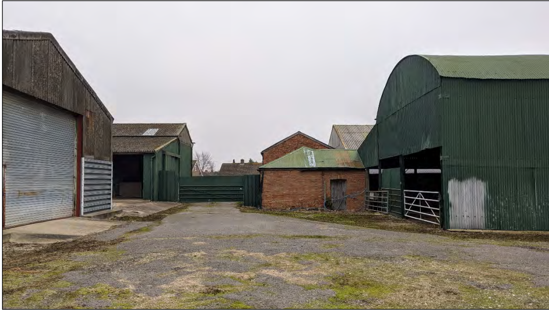
Photo 5 Disused agricultural buildings in Parcel 1
