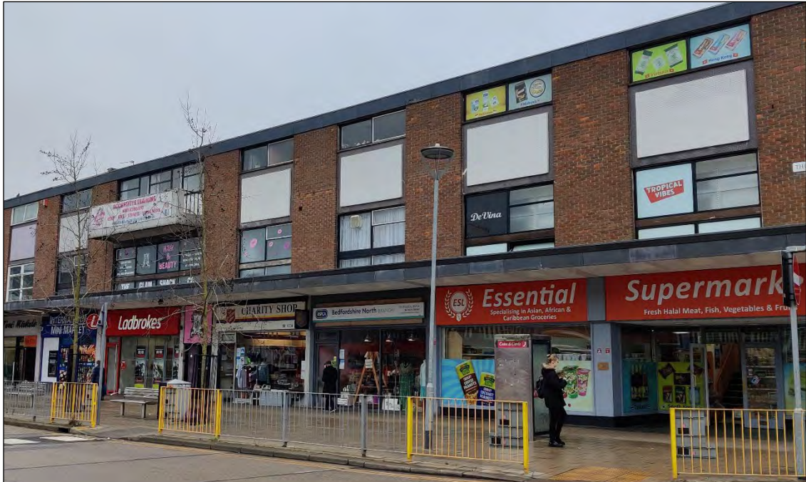
Photo 7 Retail units in the north of Parcel 4, taken from the bus station
