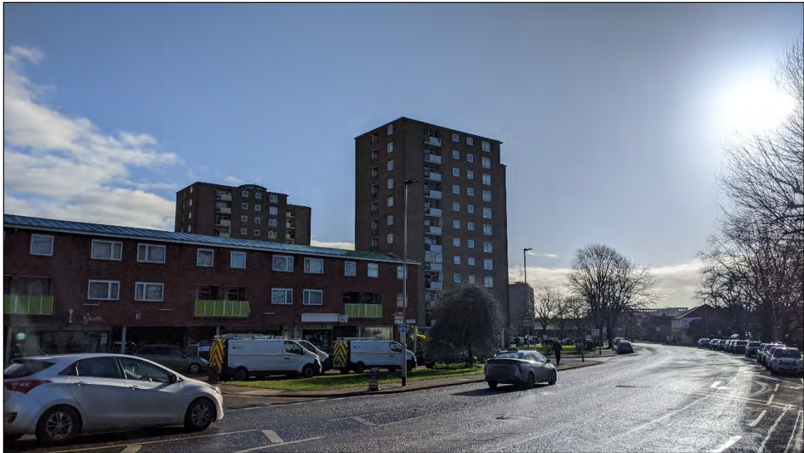
Photo 4 Greyfriars shops and tower blocks
