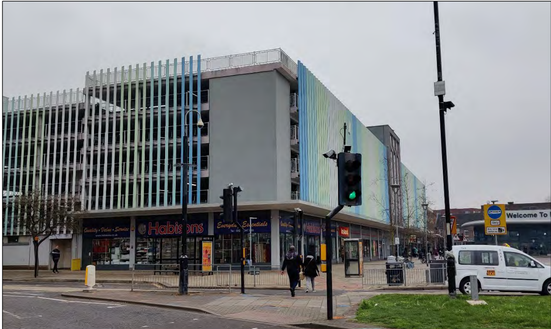
Photo 5 Multi-storey car park and retail units in Parcel 3
