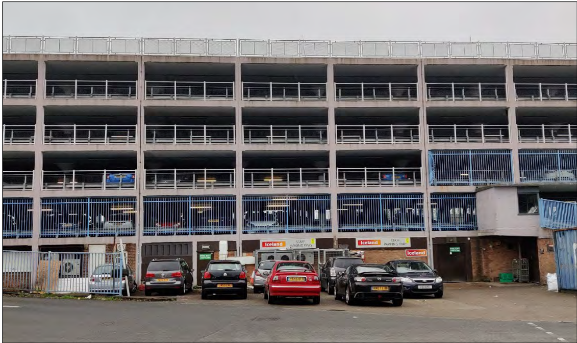
Photo 6 Multi-storey car park, taken from the junction of Brace Street and Gwyn Street
