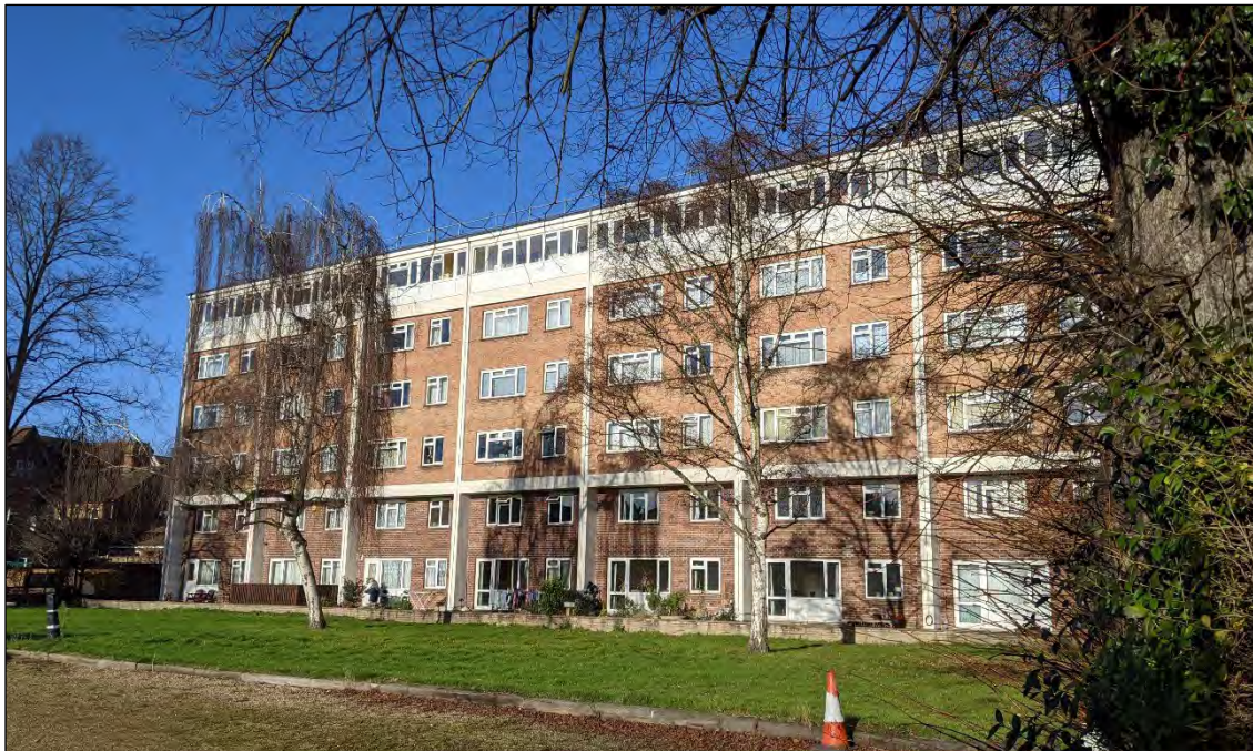
Photo 1 South façade of tower block on the west of the Site
