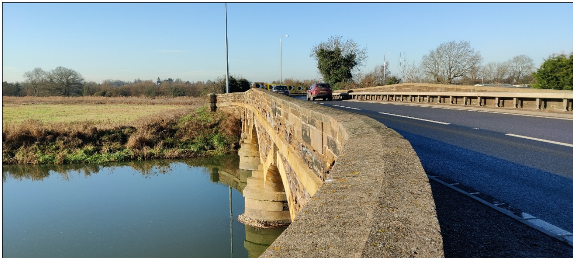
Photo 5. View of the bridge from the bridge
