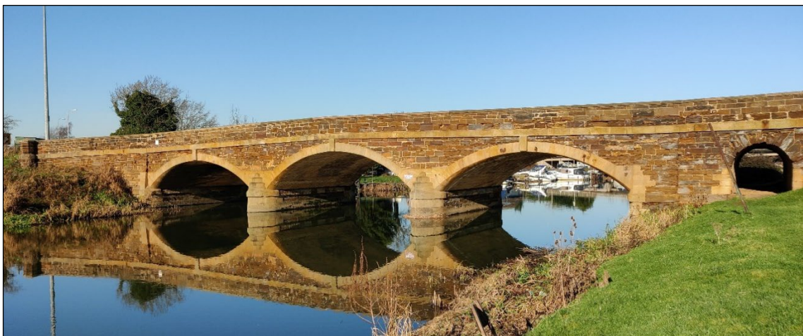
Photo 1. View of Tempsford Bridge from the south
