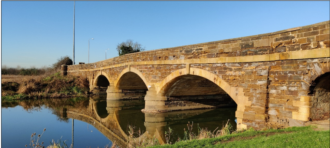
Photo 3. View of Tempsford Bridge
