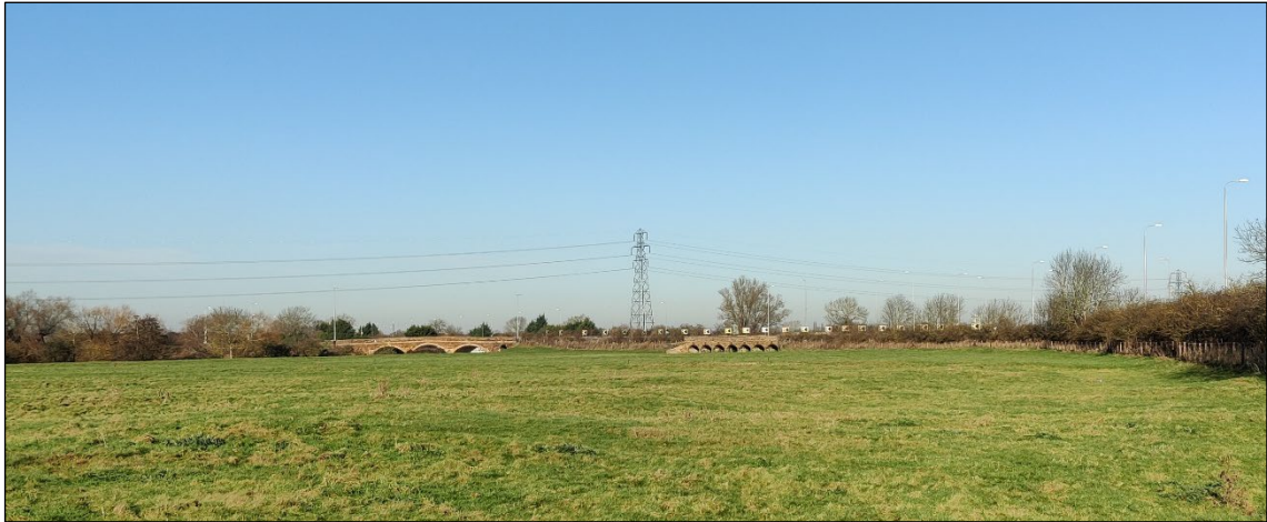
Photo 4. View of Tempsford bridge and eastern flood bridge from the south
