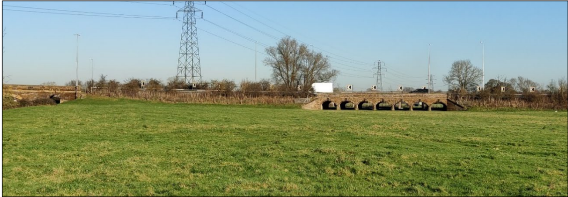
Photo 2. View of flood bridge to east of Tempsford Bridge
