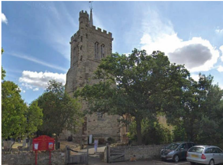
Looking south-east towards the Parish Church and Tower
