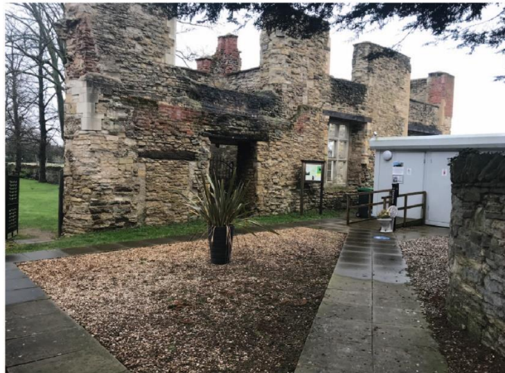
Looking south-east at the extant remains of Hillerdon Mansion
