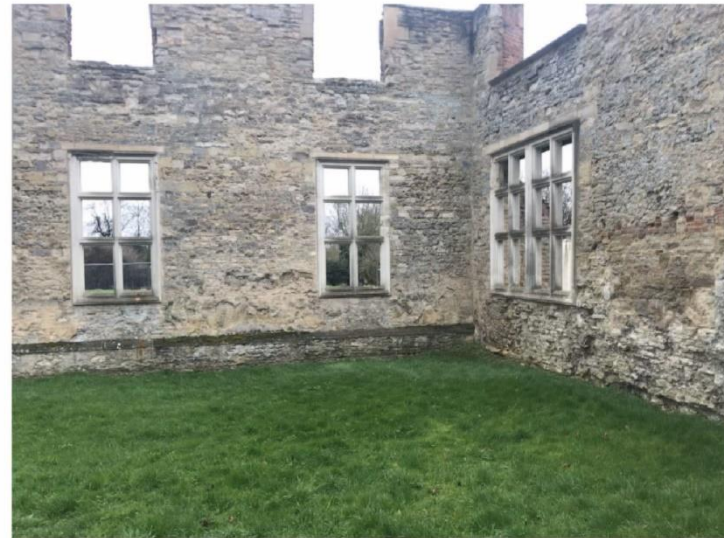
Looking south-west at the southern elevation of Hillerdon Mansion
