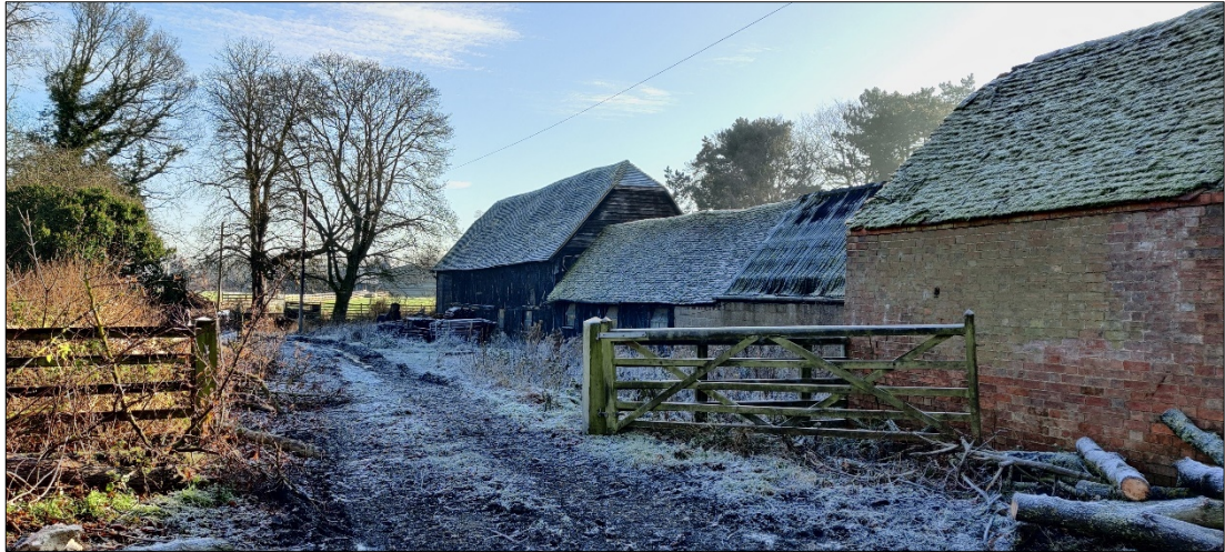
Photo 4 View of the rear of the Stable Block
