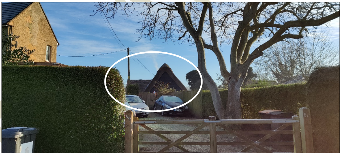
Photo 7 View of the roof of 52 Green End
