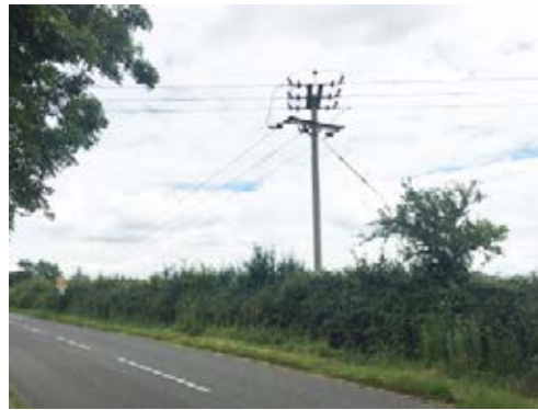
View 1 - View looking south-east towards site along Wood End Lane
